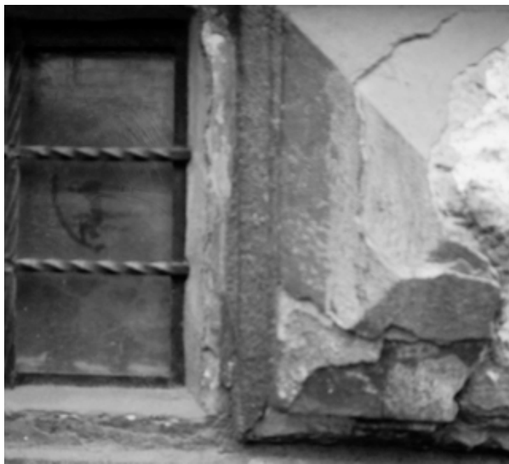
Figure 4: Wall Detail . Andrásy út, Budapest. Author's own (30 Dec 2014).
